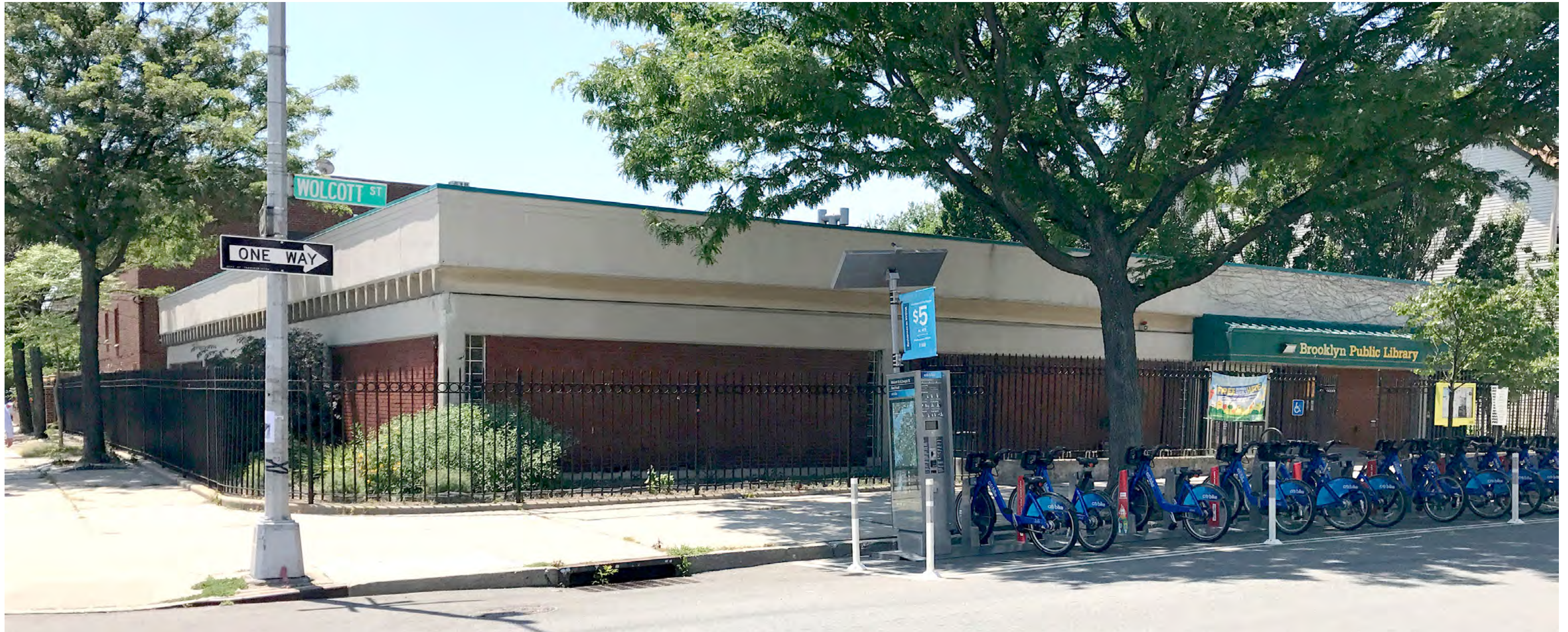
View from Corner of Wolcott Street & Dwight Street
